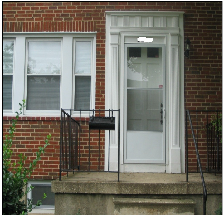
Middle of Group Covenant Compliant Home 2 Original Design Fluted Pilasters and Plinth Blocks on each side, 6 Fluted Teeth and Cross-head above Door and Double Hung Windows
