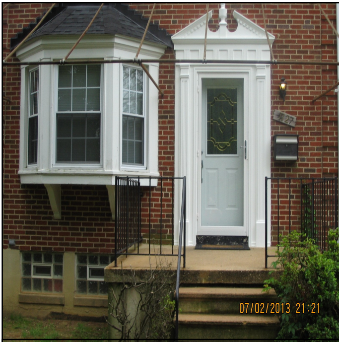
End of Group Covenant Compliant Home 2 Original Design Fluted Pilasters and Plinth Blocks on each side, 6 Fluted Teeth and Acorn Pediment and Crosshead above Door, And Double Hung Windows
