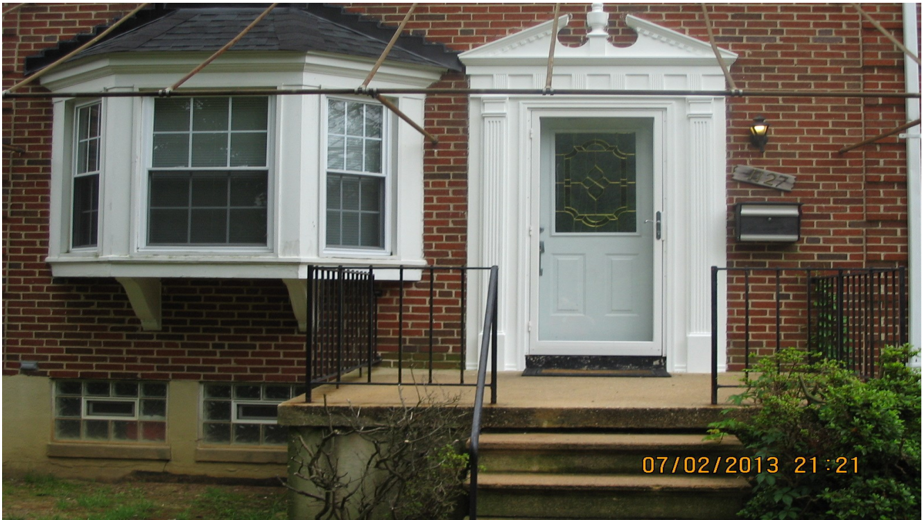
End of Group Covenant Compliant Home With Original Design Fluted Entrance Door Pilasters and Plinth Blocks, 6 Fluted Teeth and Acorn Pediment above Door and Double Hung Bay Windows
