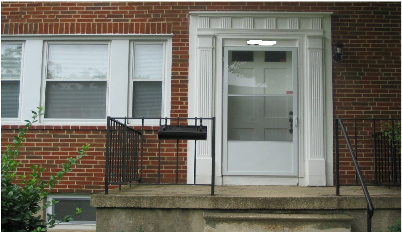
Middle of Group Covenant Compliant Home With Original Design Fluted Entrance Door Pilasters and Plinth Blocks, 6 Fluted Teeth and Crosshead above Door and Double Hung Win-
