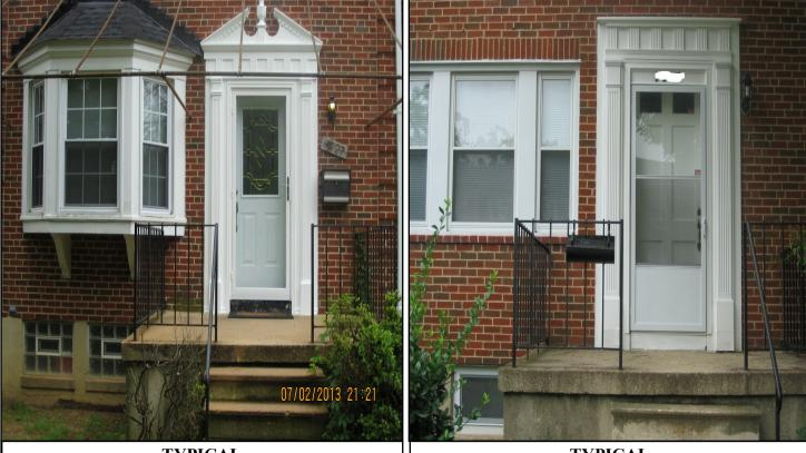
TYPICAL End of Group Covenant Compliant Home Front Entrance Door Trim Two Original Design Fluted Pilasters and One Plinth Block on each side, Acorn Pediment above Crosshead, Standard Crosshead with 6 Fluted Teeth.
